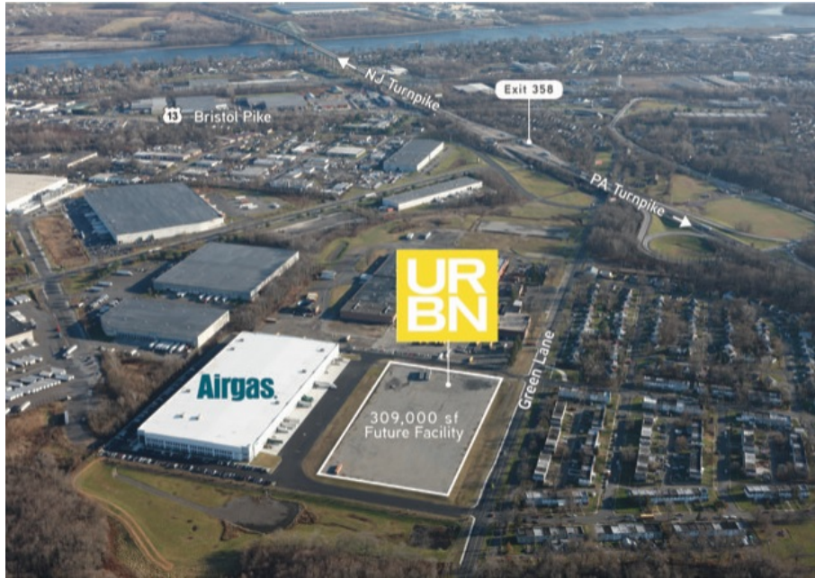
Aerial of the future 309,000-square-foot warehouse at Bristol Commerce Center in Levittown, Pennsylvania. Image credit: Colliers International
